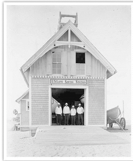
A community where the past protects our future.....
