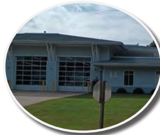
Public Infrastructure and Services
