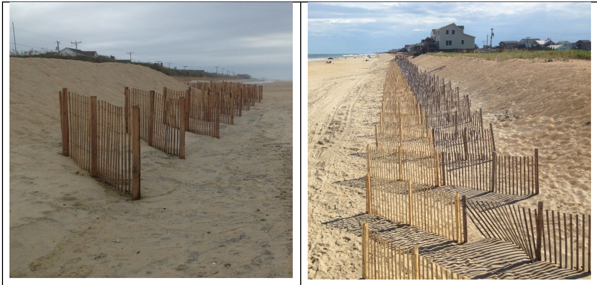
Figure 3. Examples of sand fencing placed between Stations 188+69 and 150+00 and 6+50 and 1+00 in Kitty Hawk. The photograph on the left shows sand fencing placed at the toe of the dune and the photograph on the right shows sand fencing placed in line with existing sand fencing.
