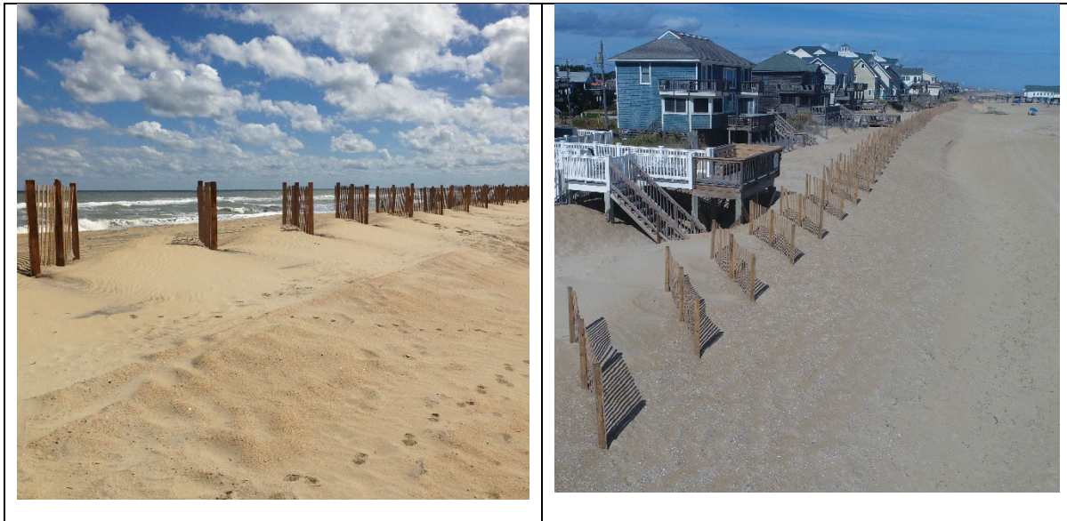
Figure 4. Examples of sand fencing placed between Stations 150+00 and 6+50 in Kitty Hawk.
